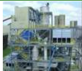
AEP Mountaineer US - 58 MWth Chilled Ammonia, coal
