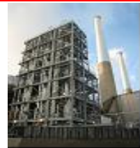
EDF - Le Havre France - 5 MWth Adv. Amines - Coal
