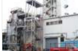
DOE/Alstom Windsor US - 3 MWth Chemical looping - coal
