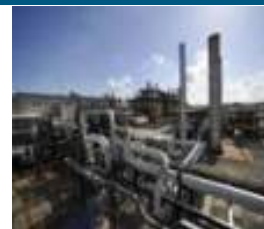
Total Lacq France - 30 MWth Oxy - Gas
