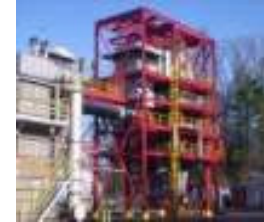
Alstom BSF Windsor US - 15 MWth Oxy - coals
