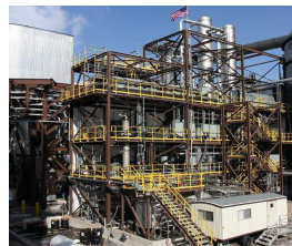
WE - Energie US - 5 MWth Chilled Ammonia, Coal
